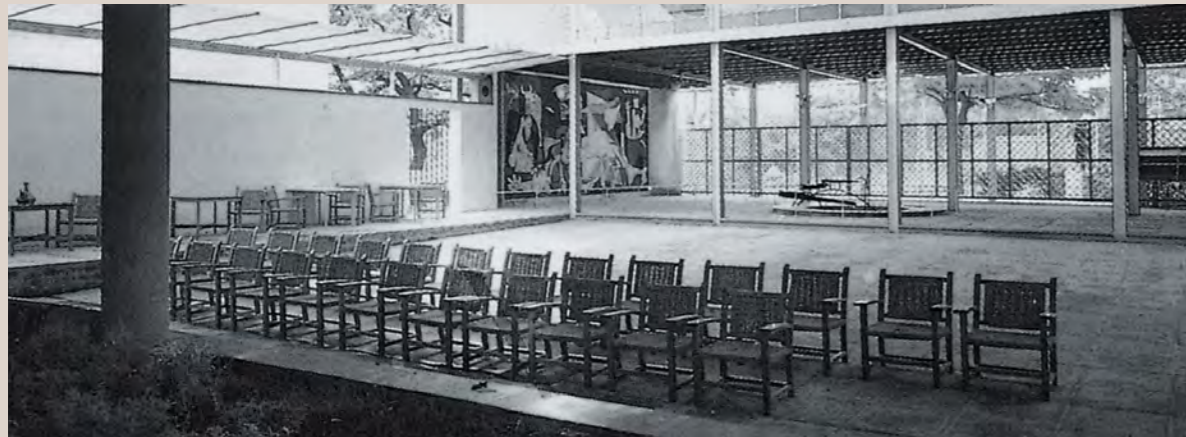
Pavilion of the Spanish Republic, International Exhibition in Paris 1937. Photo by François Kollar
